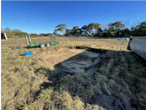
Photo 13: 7 June 2024 Area 4 looking southwest
