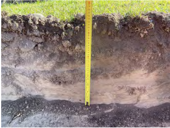
Photo 9: 7 June 2024 Area 3 side wall 350 mm excavation
