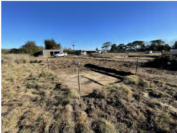
Photo 1: 7 June 2024 Area 1 looking southwest
