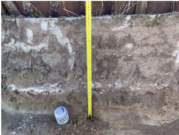
Photo 7: 7 June 2024 Area 2 western side wall – 500 mm
